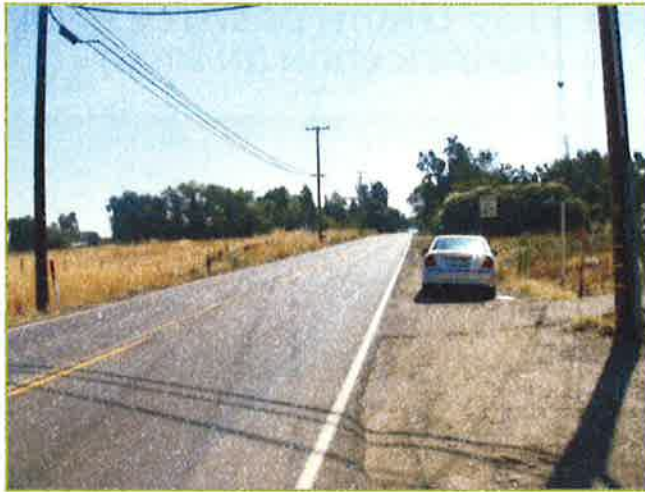
Constructing bikeways and trails in correspondence with road construction projects.
