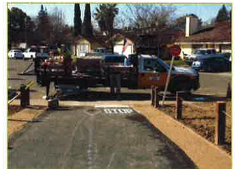
Image of trail construction in Elk Grove.
