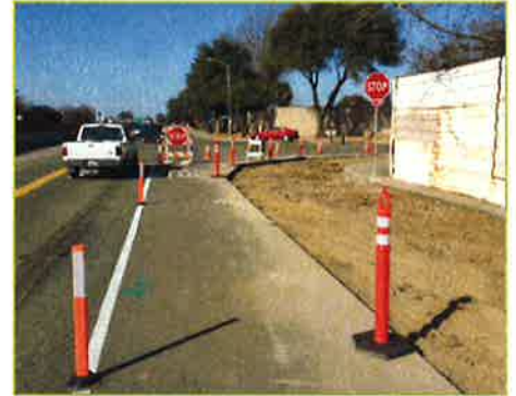
Sidewalk infill construction in Elk Grove
